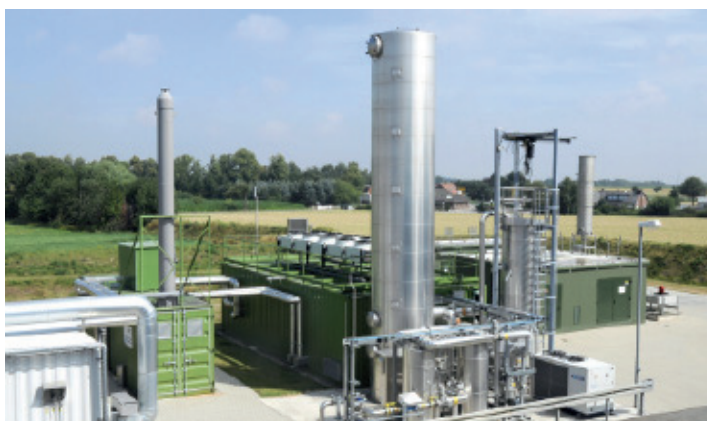
Heat-led gas upgrading process – Plant for biomethane production with pressureless amine scrubbing in Bruchhausen-Vilsen
