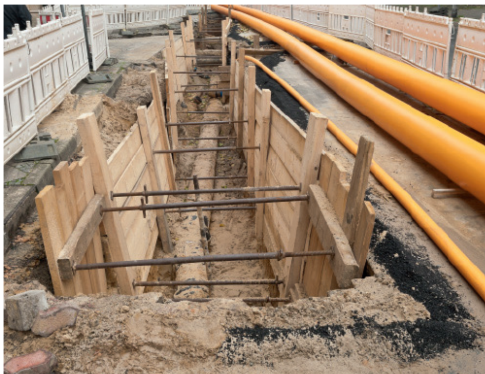
Construction of biomethane pipelines
