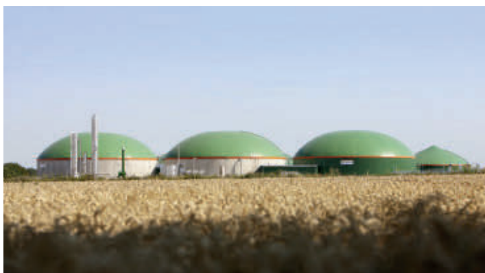
Biogas plant Vettweiß biomethane feed-in plant
