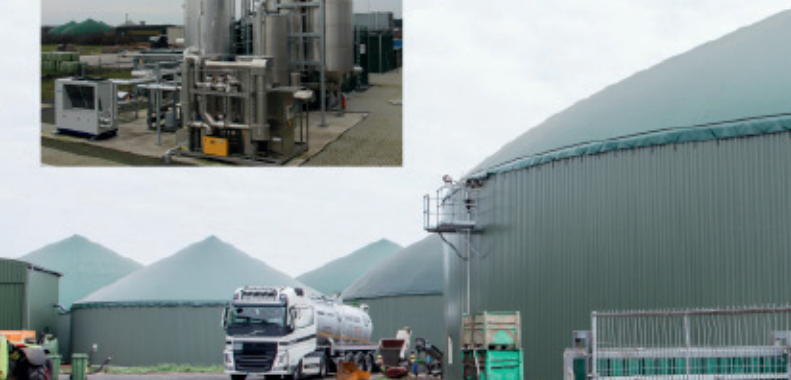
The amine scrubbing system has been proving as a reliable upgrading system
