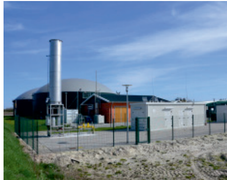
Example of a PlanET biomethane plant
