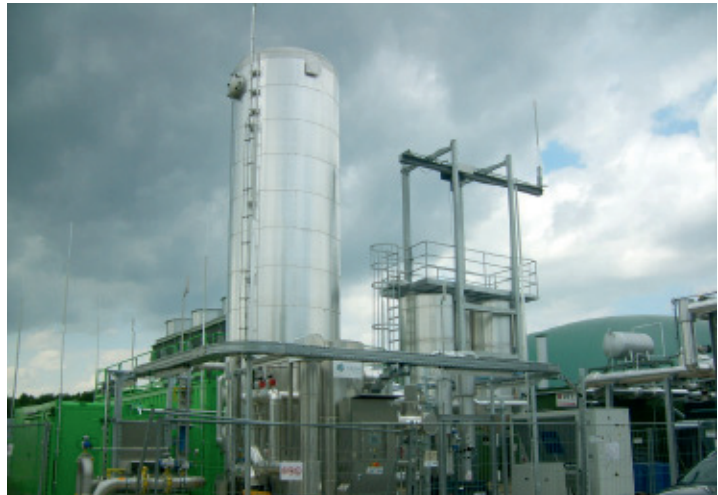
Biogas treatment plant Neudorf (Brandenburg-Germany), 700 Nm 3 per h BioMethan, amine wash process
